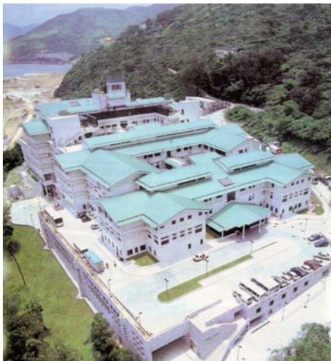
Haven of Hope Hospital (MVAC Installation)
