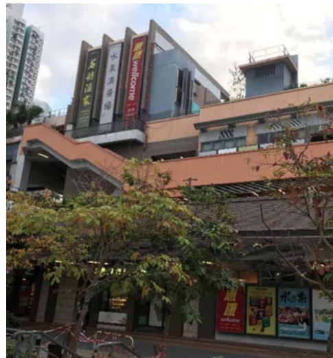
Shui Chuen O Estate (Electrical Installation)
