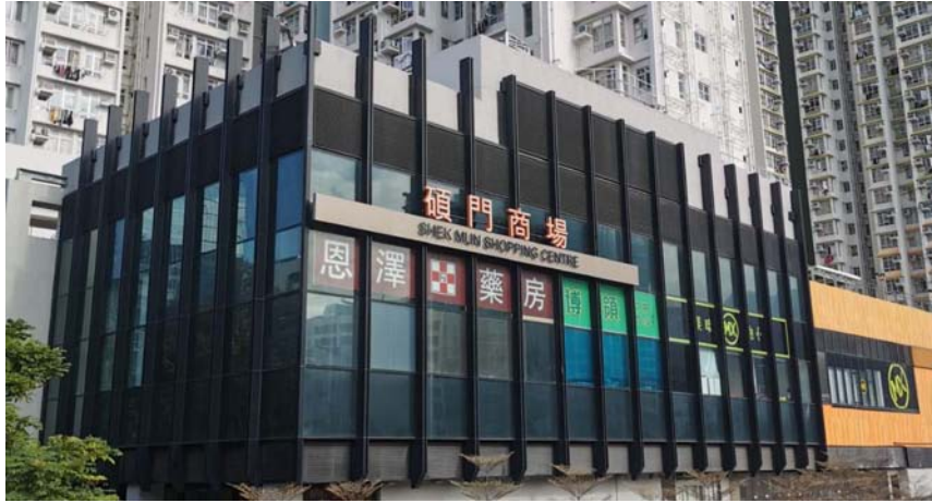
Air-Conditioning and Mechanical Ventilation Installation for Construction of Public Rental Housing Development at Shek Mun Estate Phase 2, Shatin
