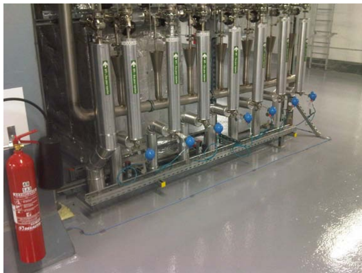
Figure 5 Installation of water sense cables on the floor near water pipes
