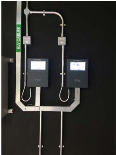
Figure 6 Two liquid leak detection monitoring panels installed inside a data centre
