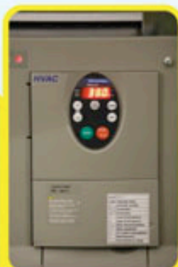
凍水泵及冷凝水泵的變速推動器 VSD on selected chilled water pump & condensing water pump for light partial load
