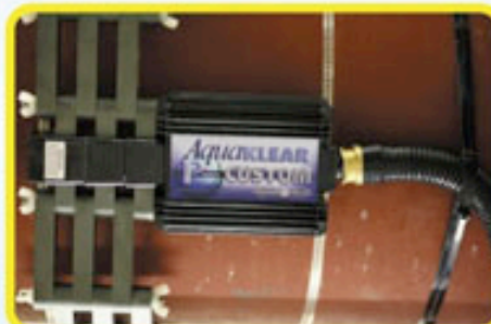
冷水機組的電磁除垢器 Electromagnetic scale remover on chiller condensing water circuit
