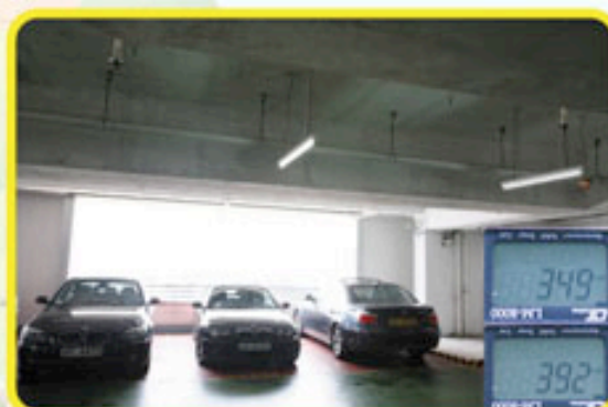
當所有燈具亮起時的比較 Lights dimmed down during daytime in carpark (note outermost row of lights turned off)
