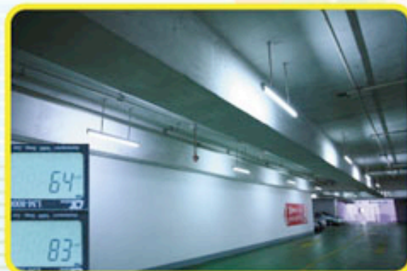
停車場內照明在日間時會被調暗 Lights dimmed down during daytime in carpark at upper lux meter reading with no visible impact (lower lux meter reading is intensity with lights at full brightness)
