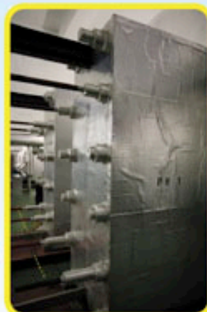
使用板式熱交換器去抽取殘餘的冷氣 Plate heat exchanger to retrieve residual cooling from chilled water circuit
