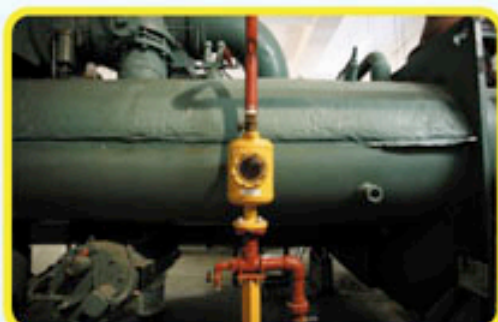
冷水機組的自動喉管清潔裝置 Automatic tube cleaning for chiller
